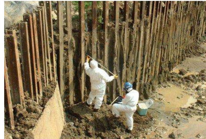
Operator protection working in the site
