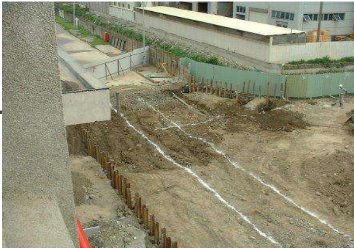
Removal of surface soils
