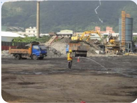
Spray to prevent dust
