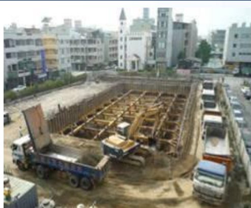
2. Install steel sheet piles
