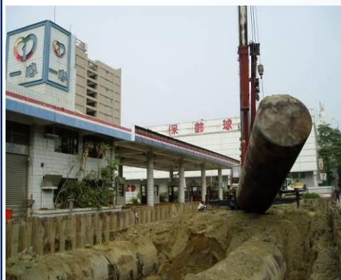
2. Remove out oil tanks
