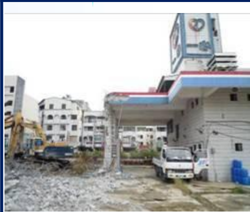
1. Tear down the building structures and gas filling islands
