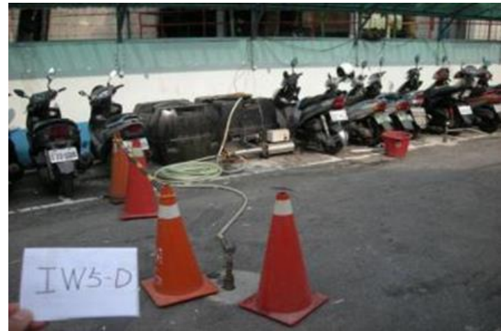
Preparation and injection of EOS solution
