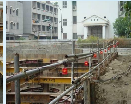
8. Fences and alarm lights
