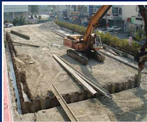
1. Install steel sheet piles
