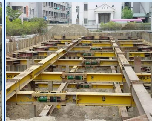
4. Install bracing structures
