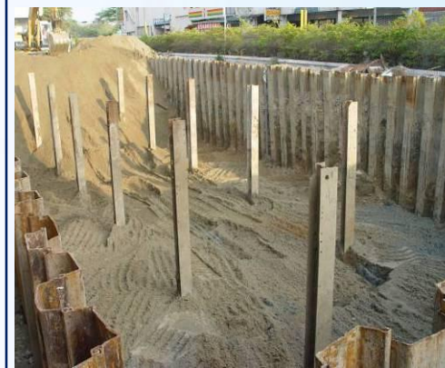
3. Install intermediate piles
