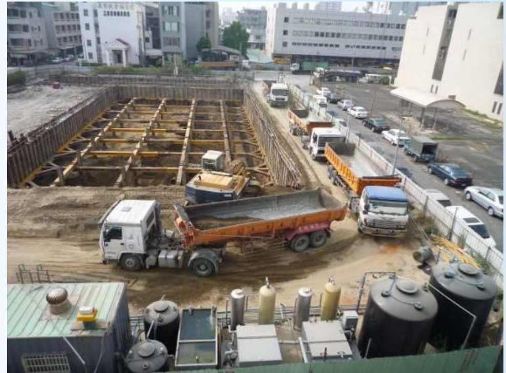
Excavation and Wastewater Treatment
