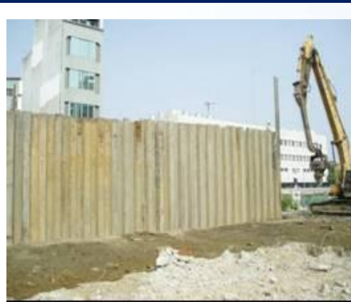
2. Install steel sheet piles
