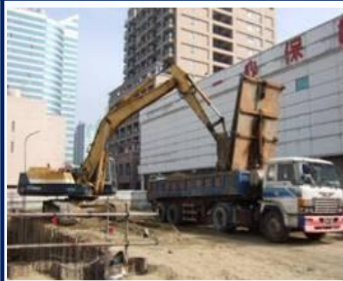
1. Tear down the building structures and gas filling islands
