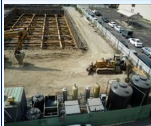
6. Relocate the wastewater treatment facilities
