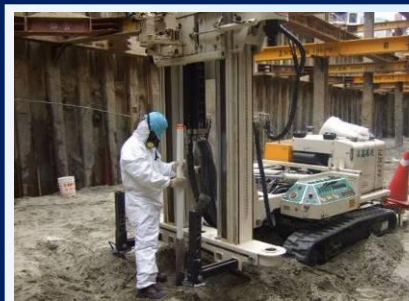
1. Injection/monitoring well Installation
