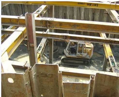
5. Excavate to 7 m bgs
