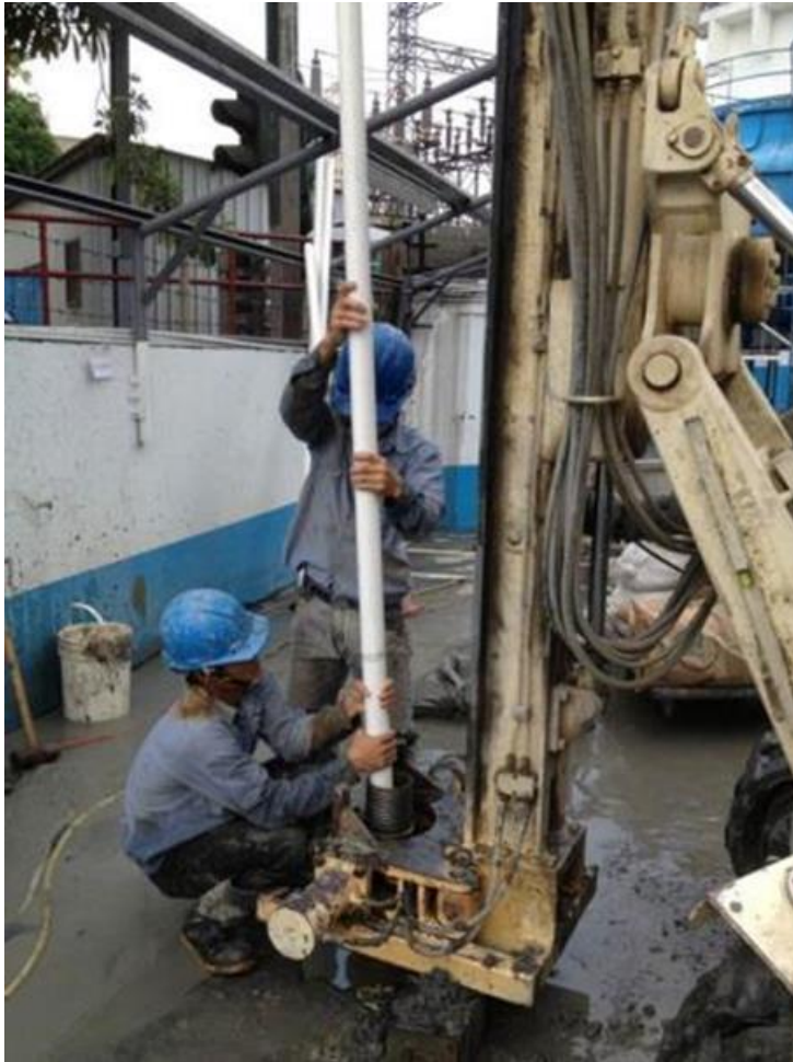
Installation of EIB injection wells
