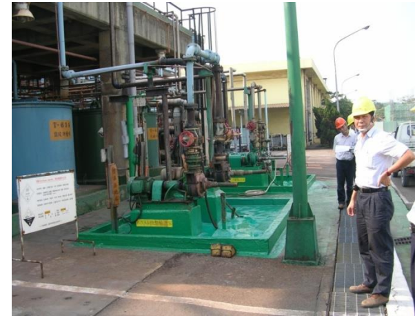
Corrosion prevention coating
