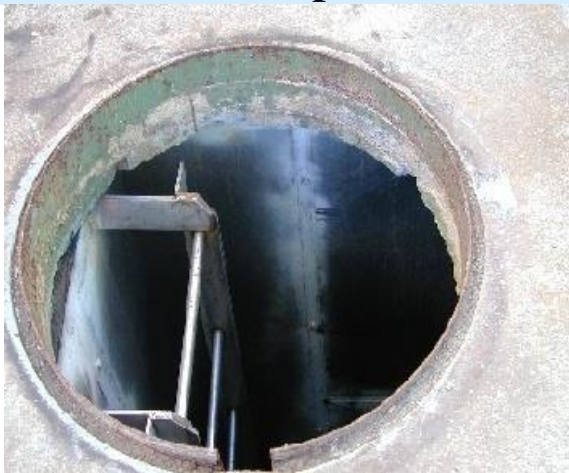
Stainless steel storage tanks
