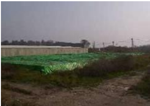
Temporary Storage Area for Soil Curettage
