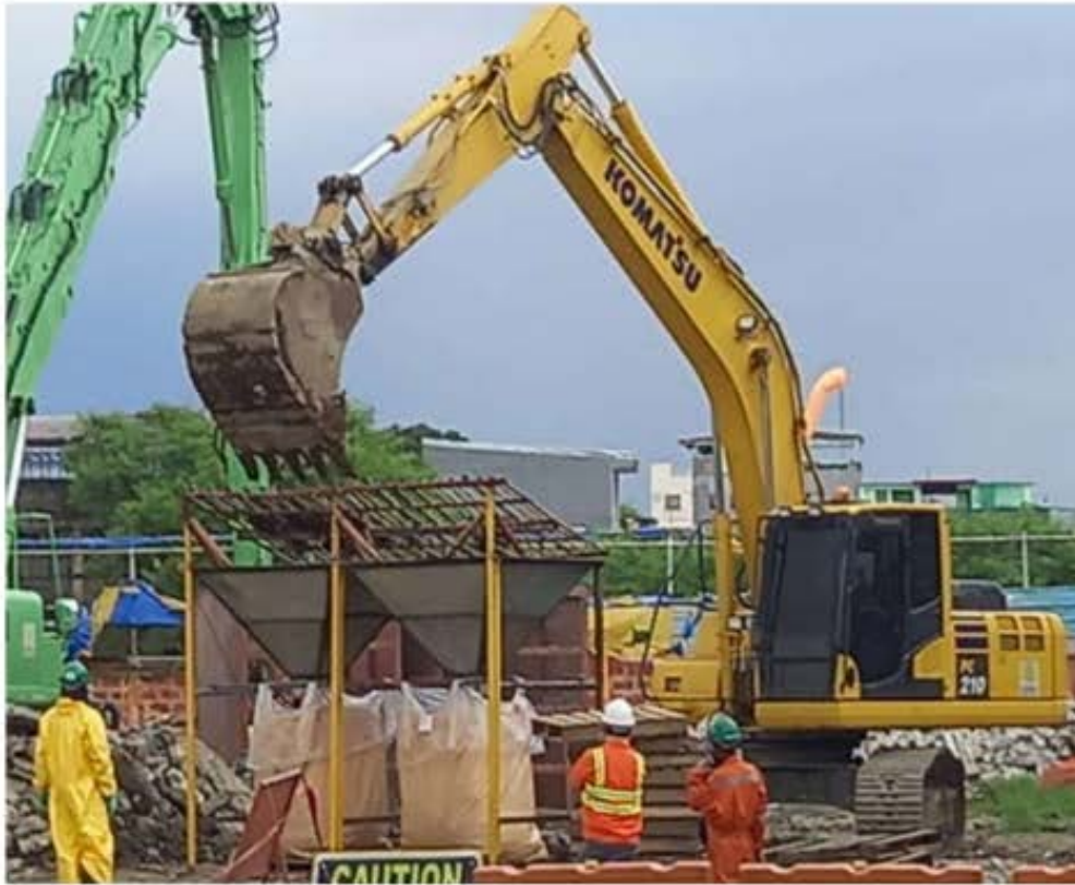
EXCAVATION, BAGGING AND TRANSPORTATION OF TONNER BAGS FROM AREA 7
